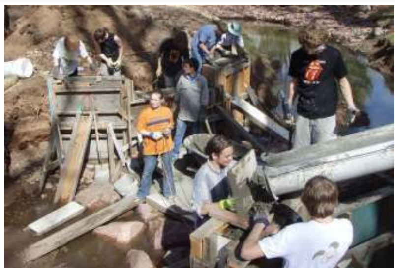
Pouring the Bridge Foundation Wing Walls.
