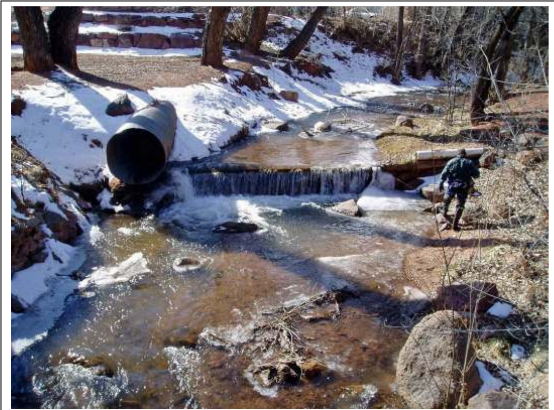
Pre-project pond diversion structure with 48" storm water culvert.
