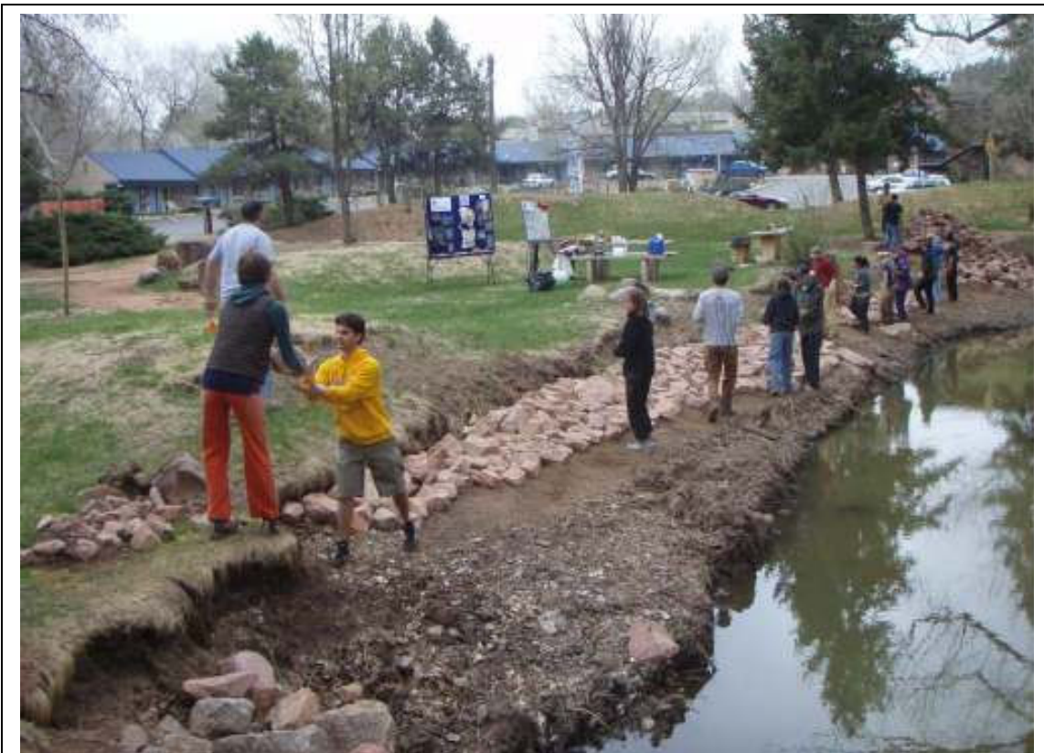
RMFI volunteers placing rip-rap along the shoreline of Shryver Pond.
