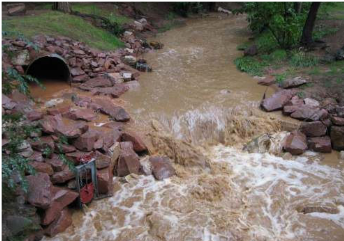
Shryver Pond Diversion Structure during the Sept 16, 2009 flood event.
