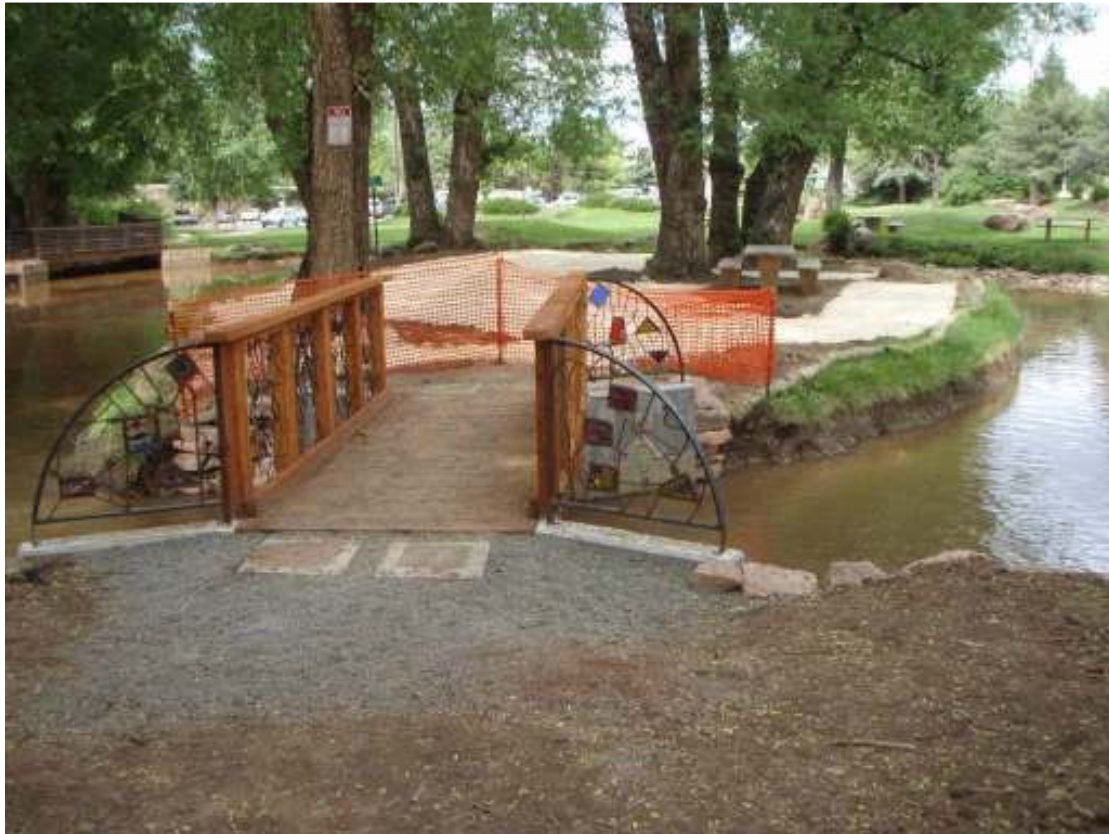
The finished footbridge constructed by high school students at Shryver Pond.
