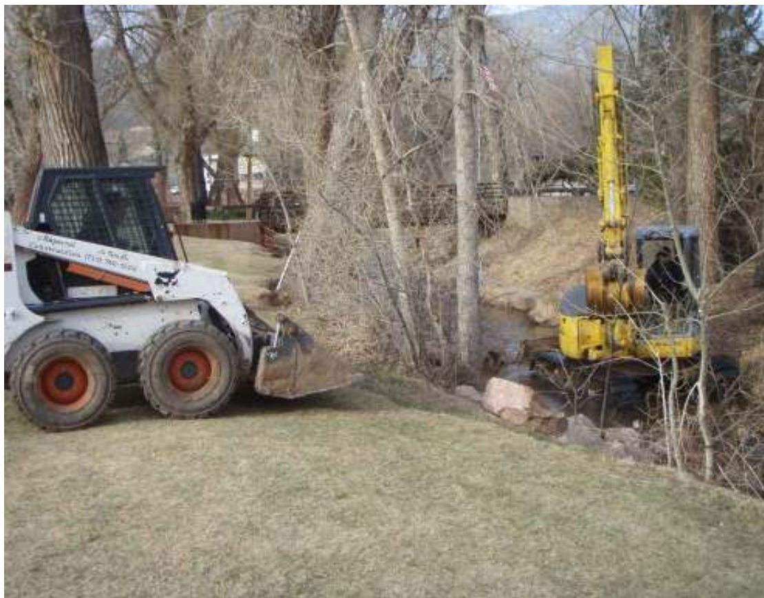
Constructing a boulder cross vane in Fountain Creek. April 2009.
