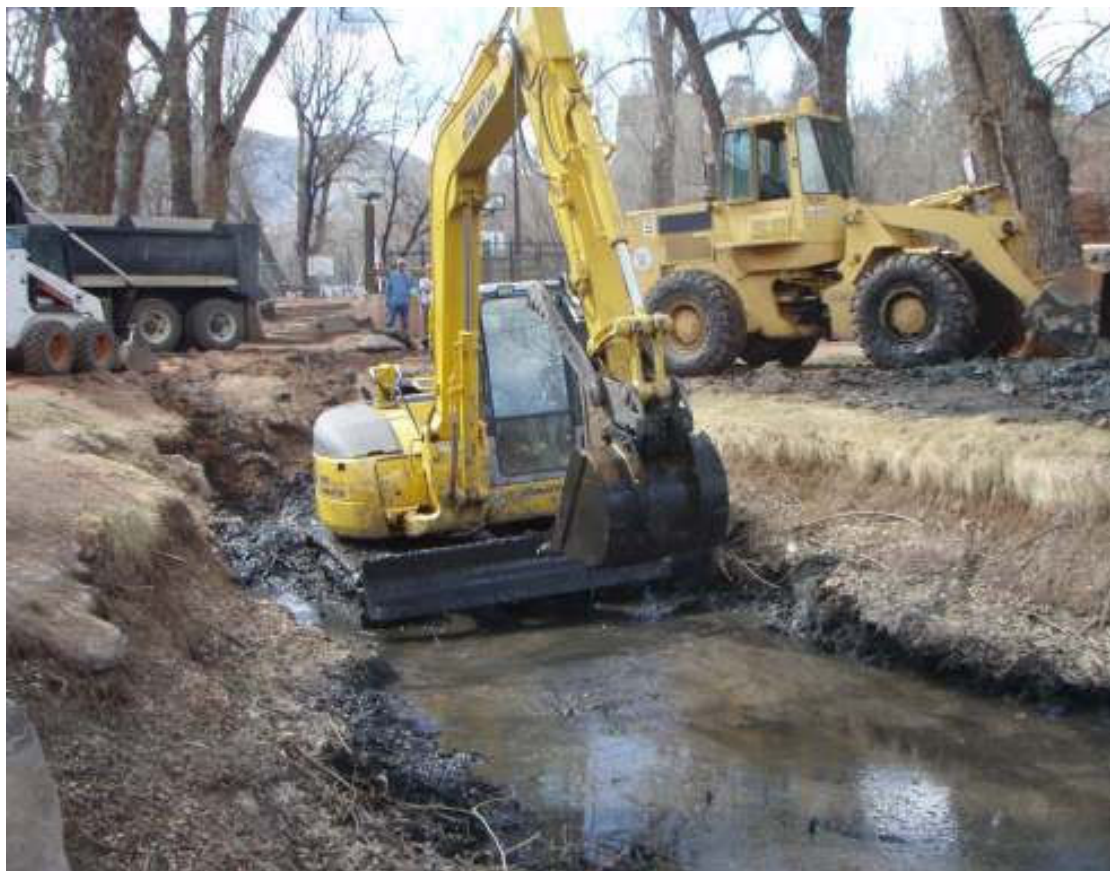
Dredging Operations in Shyrver Pond. April 2009.
