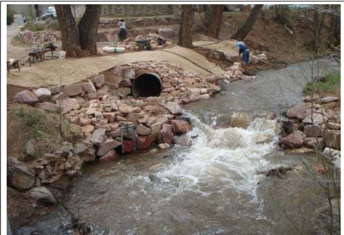
Post-project pond Dual Head-gate diversion structure with 48" storm water culvert.
